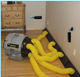
Record relative humidity and Temp in the room as well as in the insulation inside the wall.
